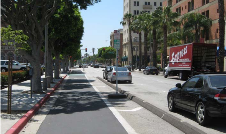
Looking west on Third Street east of Cedar Avenue; There is a driveway opening between the parking spaces and the westbound left turn lane at Cedar Avenue
