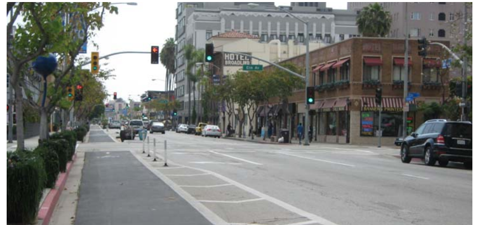
Cycle track on the north (left) side of Broadway and a modified signal at Elm Avenue
