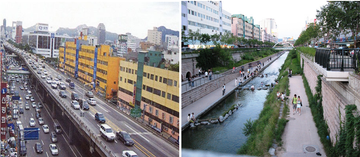
Figure 3. The Cheong Gye Cheong River in Seoul, South Korea before daylighting (left) and after (right).
