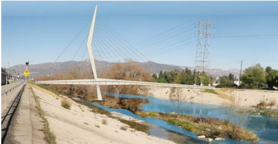
Figure 5: Future La Kretz Crossing over the Los Angeles River. 266
