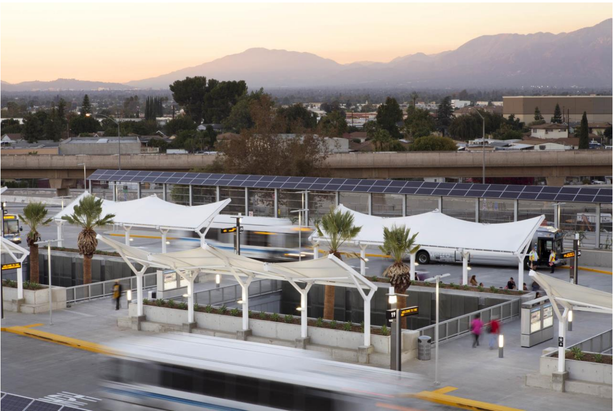
El Monte Station
