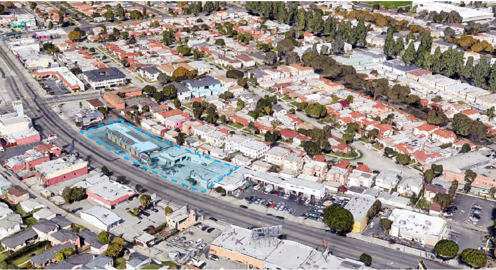
BUILDING SITE ALONG CRENSHAW BLVD
