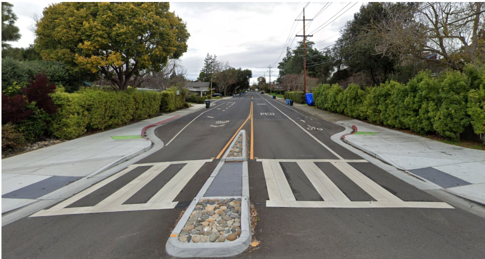
Class II bike lane and Class III sharrow on Meadow Dr in Palo Alto at a neighborhood traffic circle intersection
