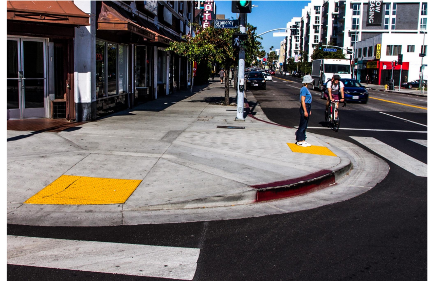
Permanent curb extensions design example
