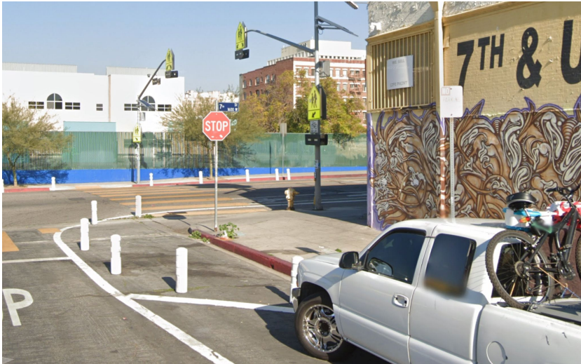
Pilot curb extensions design example
